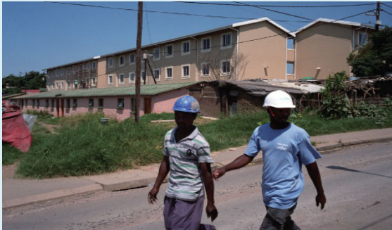
Construction of a housing project in KwaMashu, the largest poor township near Durban, South Africa (Photo credit: Africa Media Online)
