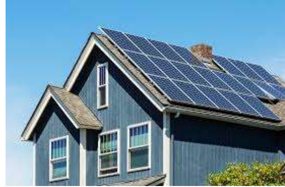
Roof-top solar panels (washingtonpost.com)
