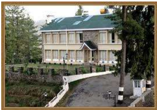
Figure 20. Circuit House in Narkanda
